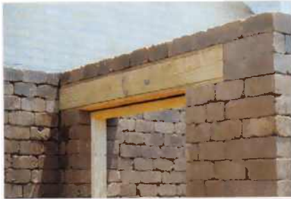
The adobe blocks (measuring 12" x 4" x 4-10") weigh 25 pounds and are dry-stacked without mortar.
