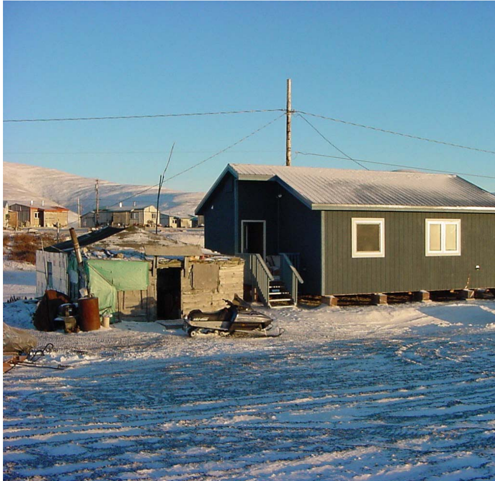
Left Old House, On the Right New House Constructed in Brevig Mission BY Kawerak HIP Crew November 14 th 2001
